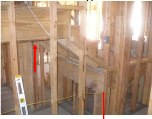
9) Missing a fireblock on the second staircase landing and the 2x riser should have a stud installed for support.
