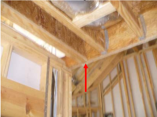
9) Missing a fireblock on the second staircase landing and the 2x riser should have a stud installed for support.
