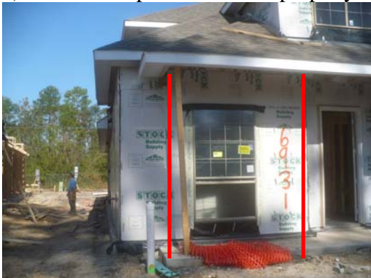
6) Permanent posts should be properly installed under the front porch beam.
